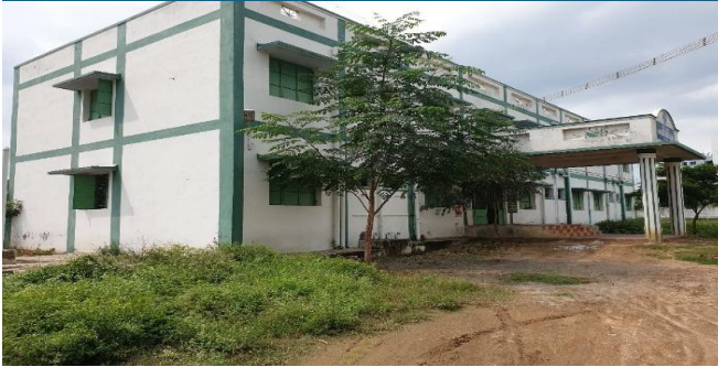
Exterior before retrofit: overgrown grounds, unmaintained façade
