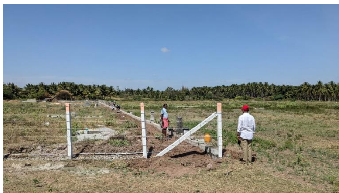
Figure 10: Site fencing work of the adjacent plot
