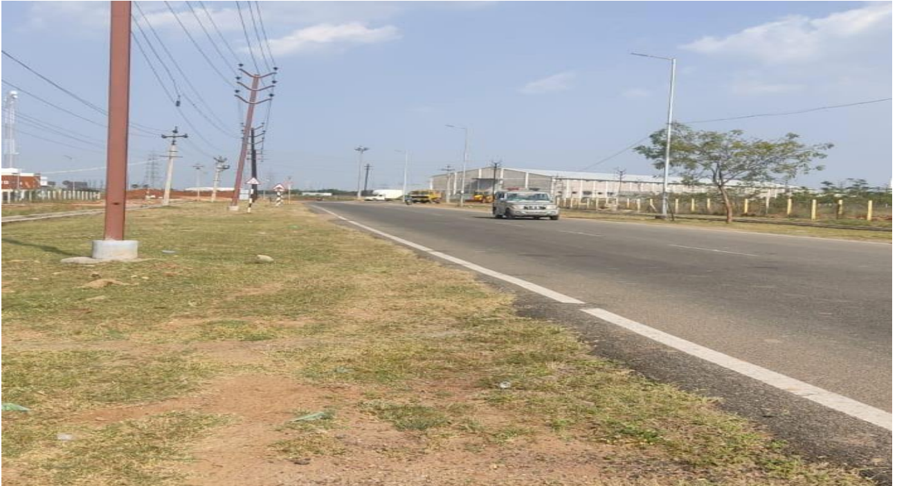
Photograph 2: Approach Road to project site towards the south side
