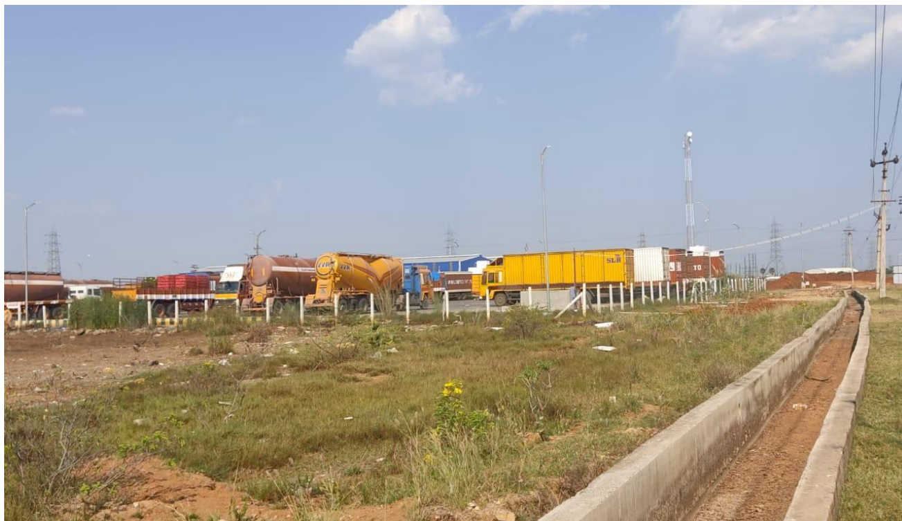
Photograph 5: View of the Site with Truck parking at the eastern plot
