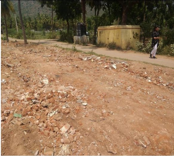
Main road widened from 10 m to 30 m
