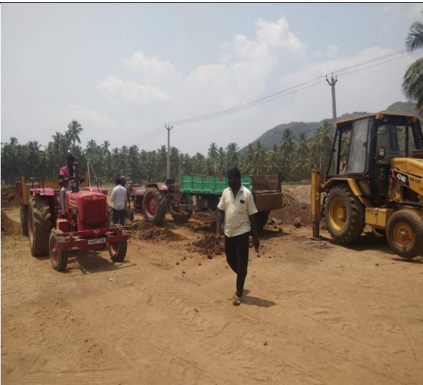
Workers involved in soil strengthening
