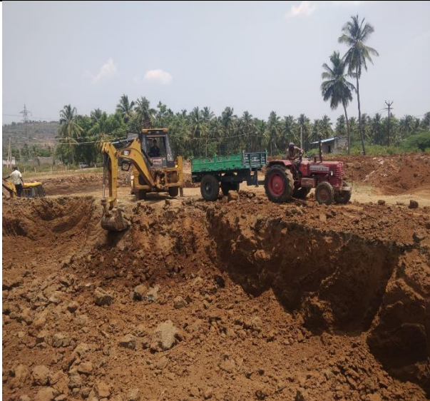
Soil stabilization and strengthening
