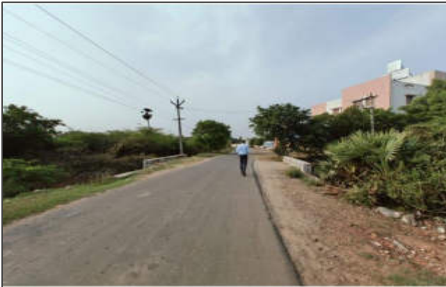
Photo 3: View of access road to project site
