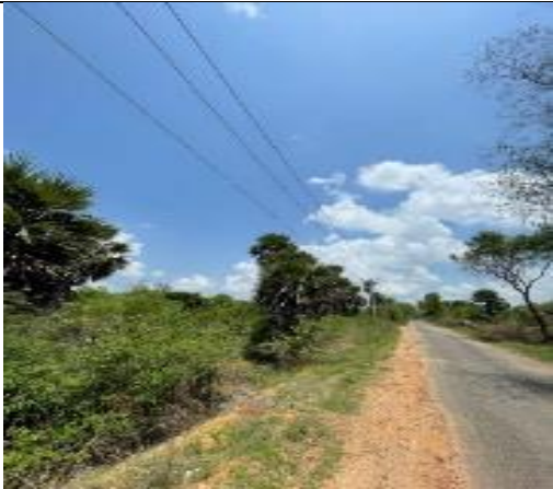
Road on north side. Unbarricaded land.
