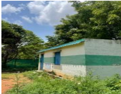
Some pre-existing temporary unused structures on site which are to be demolished.
