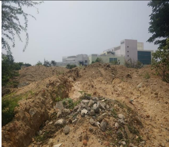
Earth filling activities
