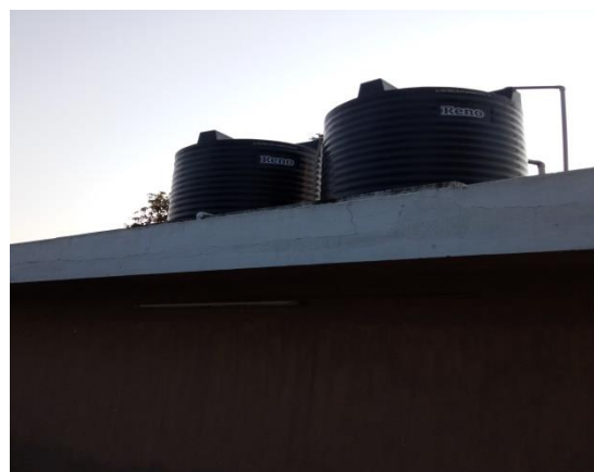
Overhead Tank at the site
