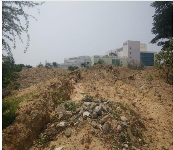
Earth filling activities
