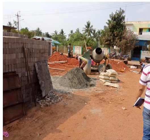
Construction work at site
