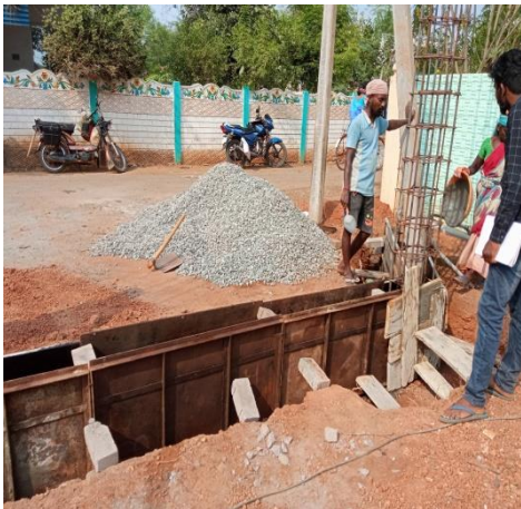
Construction work at site
