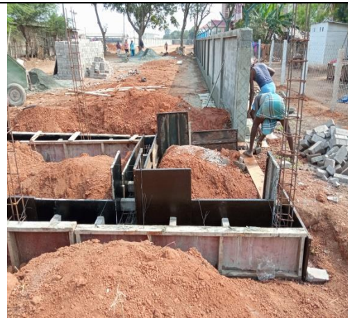
Construction work at site
