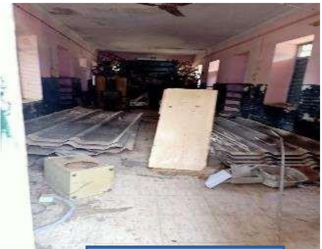
Asbestos sheets stored at site
