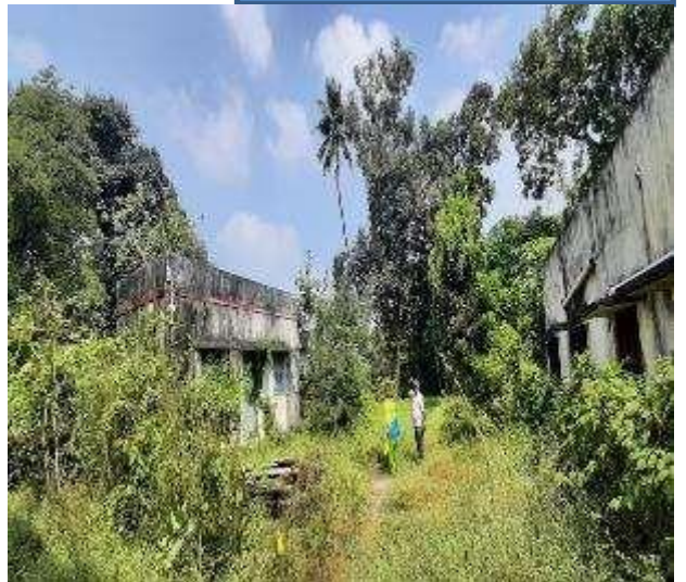
Old buildings in project site
