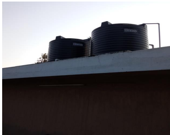
Overhead Tank at the site
